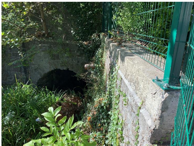
Figure 3-7: Dry Arch at the Western End of the Existing Road Bridge
