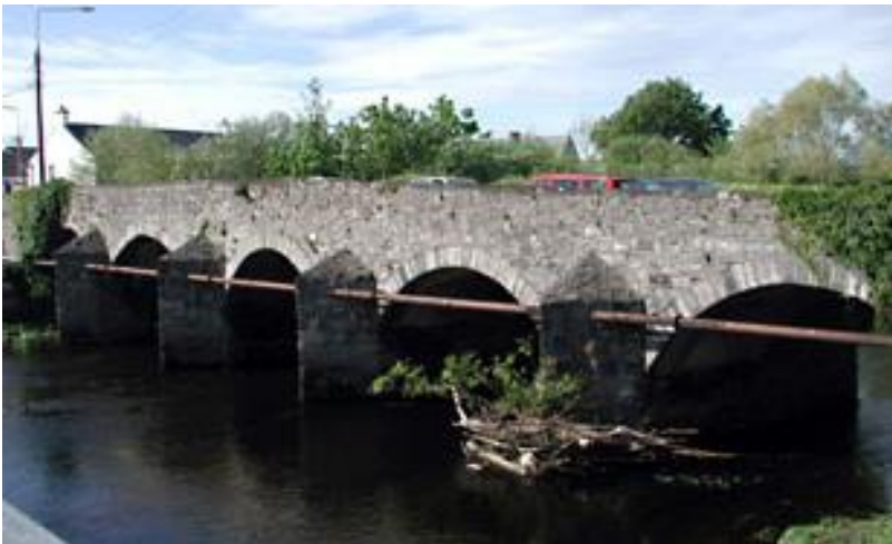
Figure 1-2: Elevation of South Western Side of Existing River Liffey Road Bridge
